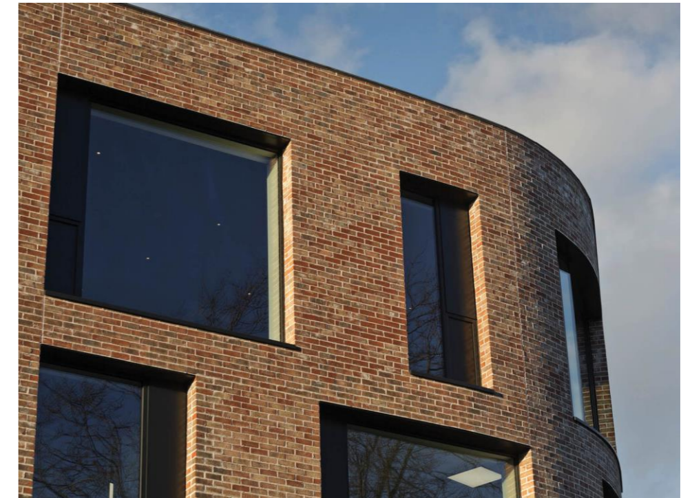
Deep reveal to windows in brick
